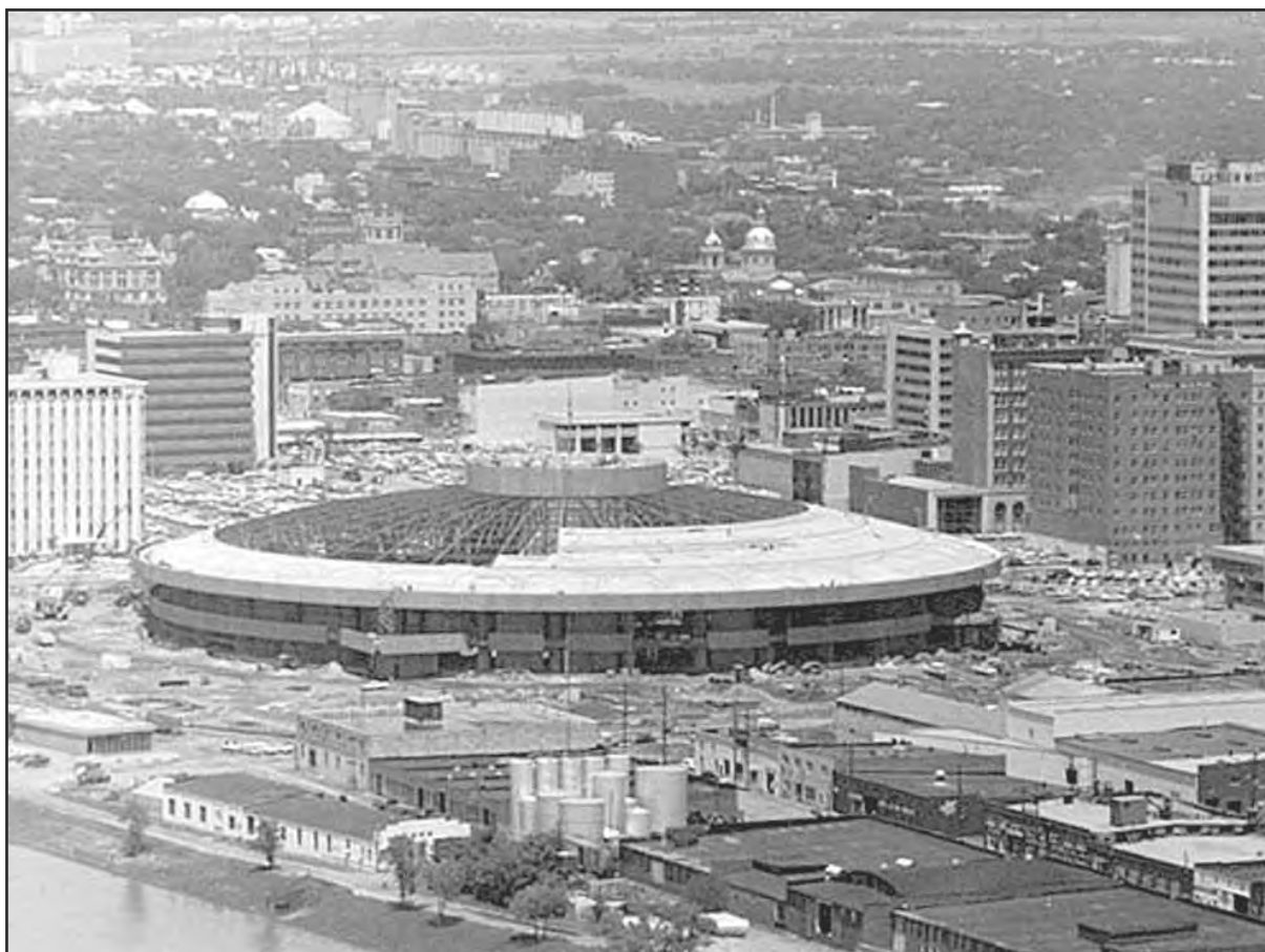
THE SAUCER HAS LANDED: This 1968 photo shows Century II under construction. Note the many industrial and commercial buildings in the foreground, all of which were cleared out in urban renewal efforts to beautify the riverfront.
